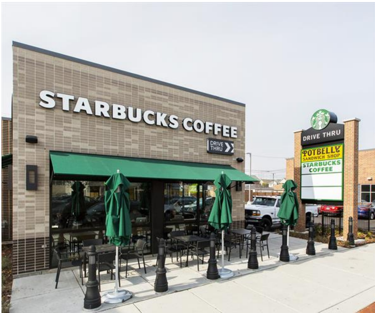
3636 North Western Avenue located in Chicago
